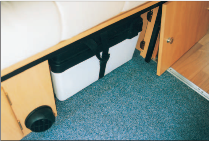
Meaty 110 amp hr leisure battery slides out from under the settee in its own container for easy checking of the electrolyte level.
