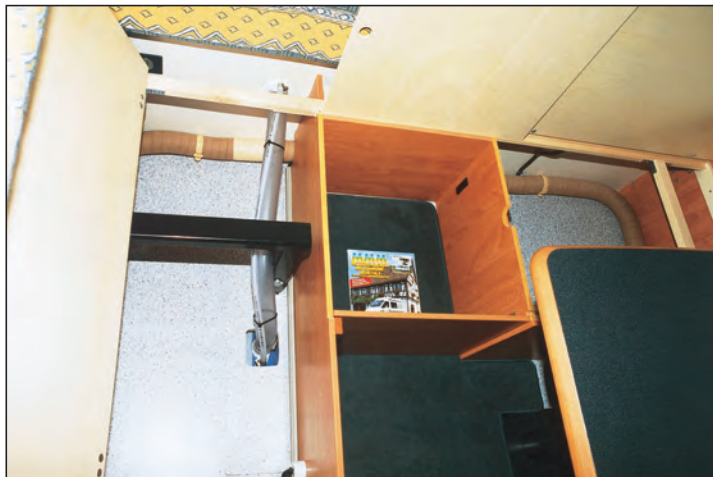
With water tanks etc underfloor, the underseat lockers are usefully empty (apart from heater ducting).
