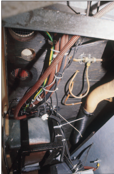
Hot-air ducting running under the 'van – not a great idea, I would have said.
