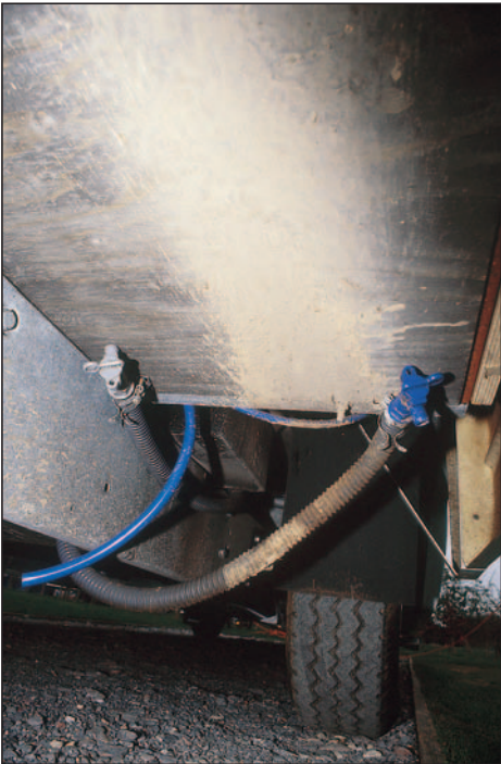
Located under the offside rear, the drain hoses and taps (for fresh and waste water tanks) are extremely awkward to reach and operate.
